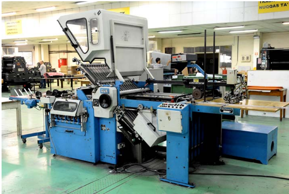
❖ Photo 6: The New Folding machine installed in 2009.
